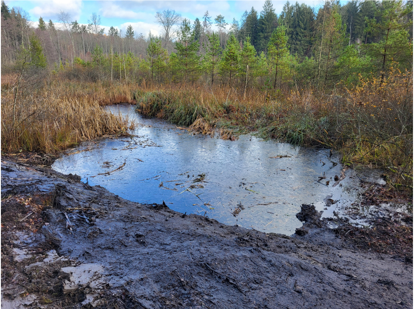
Fig. 52: The original pond 2 was deepened and simultaneously enlarged. The excavator spread the dug-up sludge along the shore.
